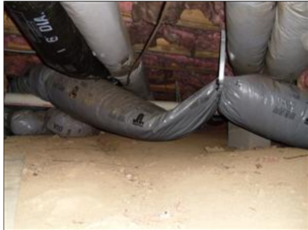
6.3 Picture 2 crush return duct
