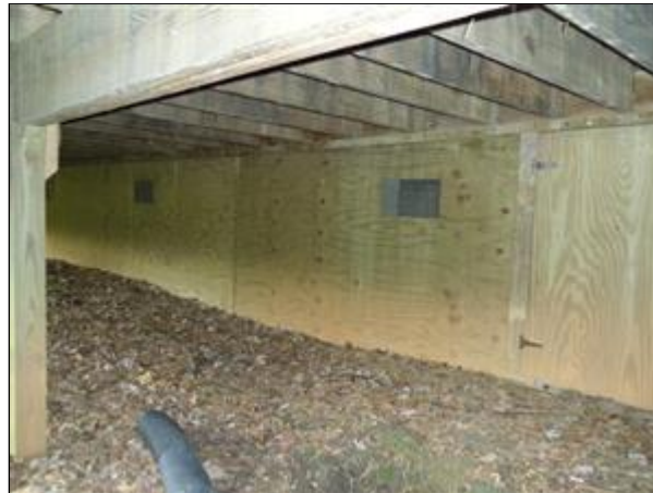
1.0 Picture 1 wood wall of foundation
