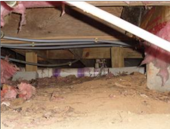
1.6 Picture 1 crawlspace under the women's bathroom
