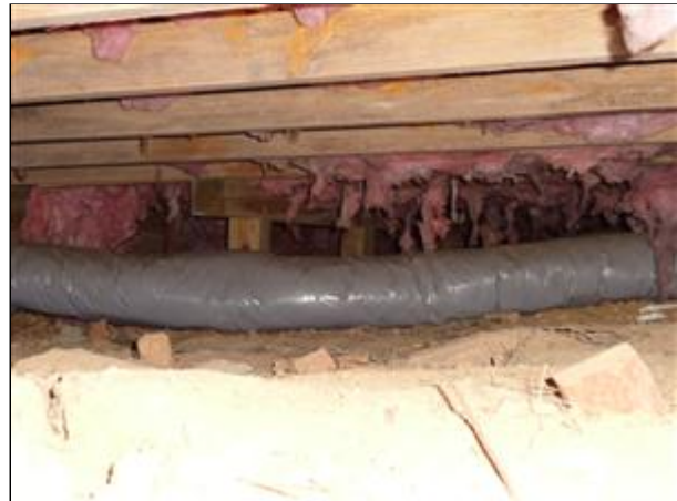
1.6 Picture 2 crawlspace under the kitchen
